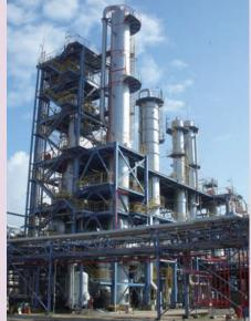
The first facility in Japan to make ethyl acetate using the ester process
